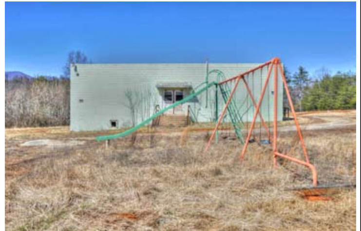
Playground at Massies Mill Elementary prior to demolition in July 2014. Photograph by Steve Trumbull.
