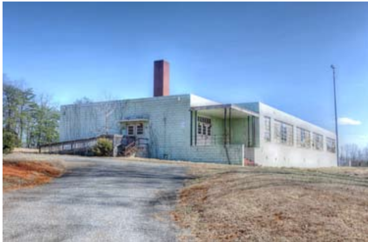
View of Massies Mill Elementary prior to its demolition in July 2014. Photograph by Steve Trumbull.
